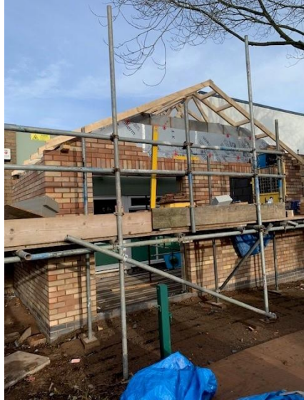
Burley Gate Primary School – Single Story Extension to the front of the school (new Library / Reception Area)
