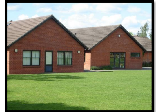
Lugwardine Primary School – Hall and Staff Room Extension
