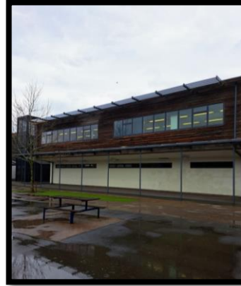
Whitecross Academy – Installation of New Canopy Structure
