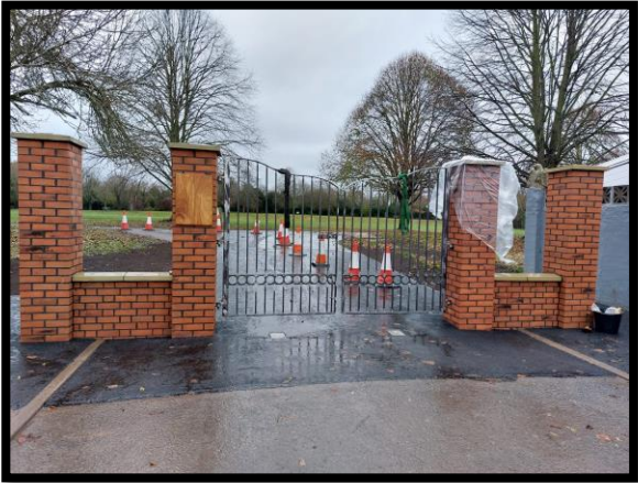
Tupsley Quarry Park – Installation of Ornate Gates into Tupsley Park
